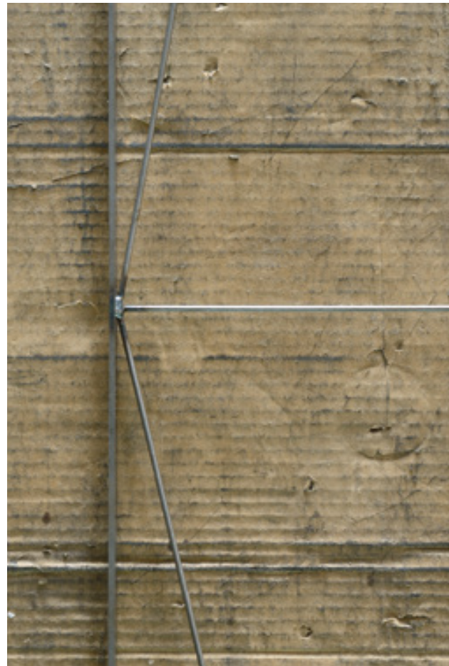
Detail of hand welding on the Opus frame.
